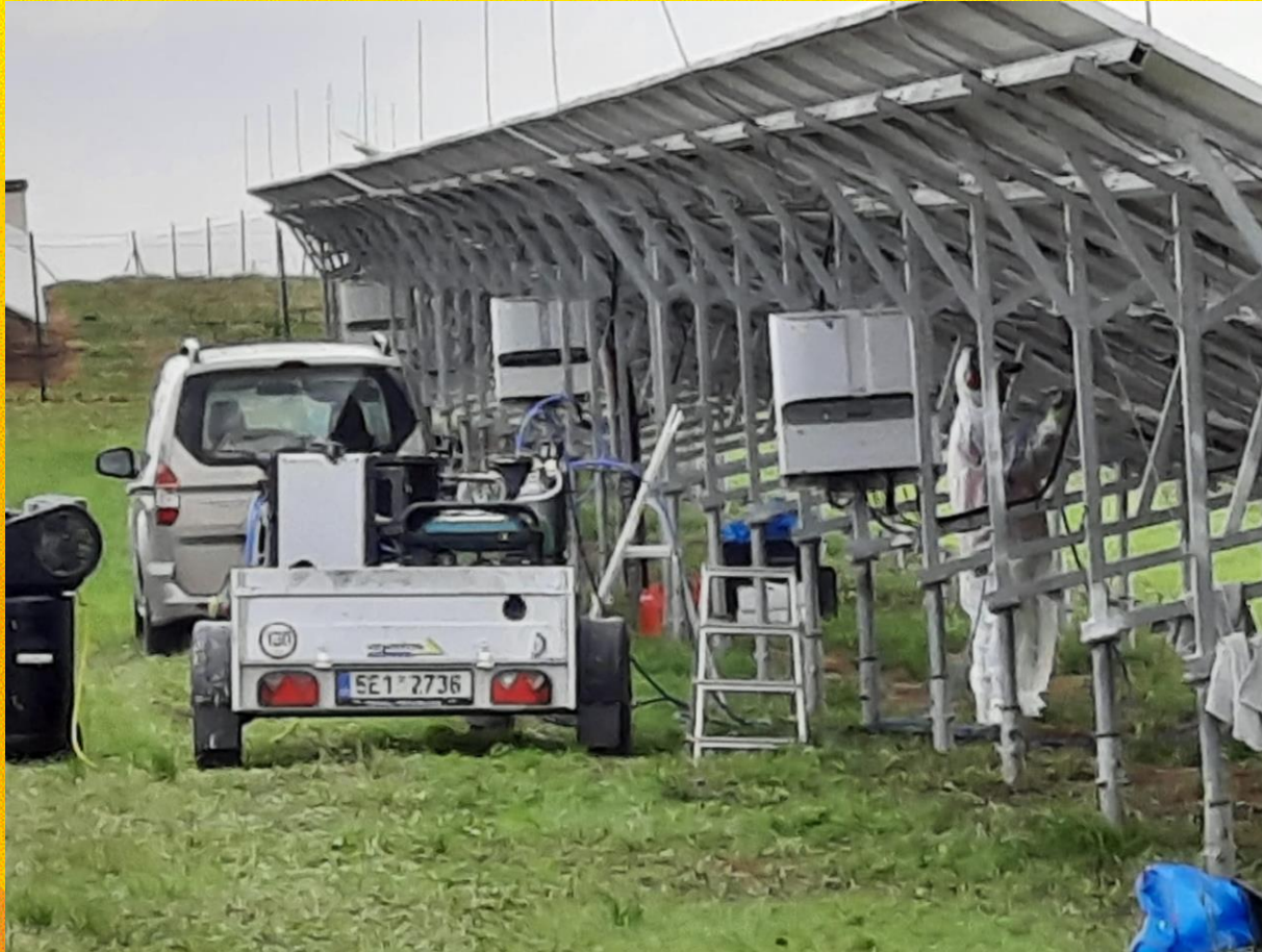
PV panel renovation equipment at 3MW PV power plant
