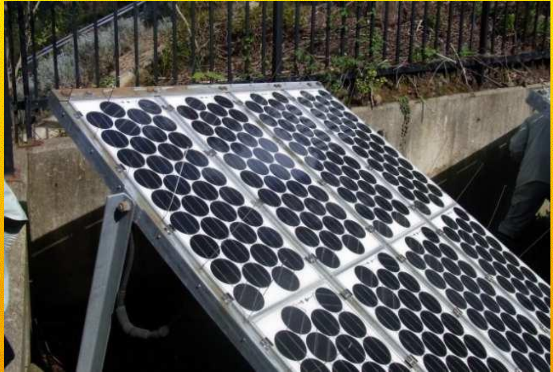
29 years old silicone laminated PV panels (Japan)
