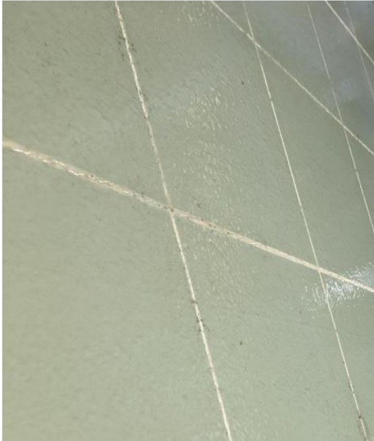
Fig. 3. Picture of renovation polysiloxane film on back side of PV panel.
