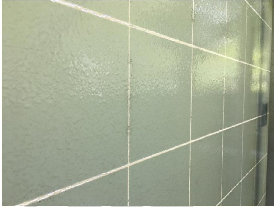
Fig. 1 Picture of renovation PDMS film on back side of PV panel.
